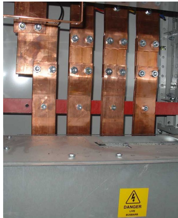
Busbars are used for ground conductors in high-current circuits.
